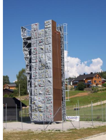
Selfstanding climbing tower made of 3D 1x1 m polyester panels
